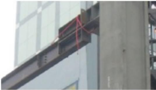
Figure 4: ‘Dog-leg’ beam connection
